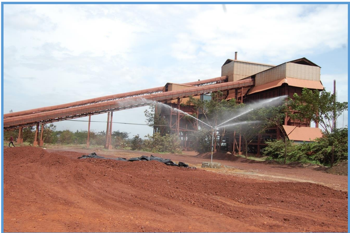
Sprinklers Installed at Mini Iron Ore Yard
