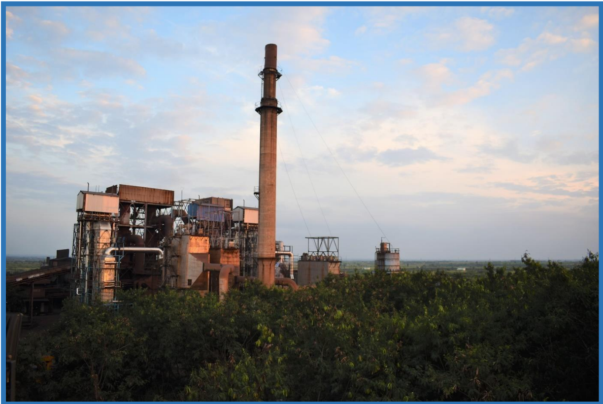
Air pollution control Equipment's with chimney
