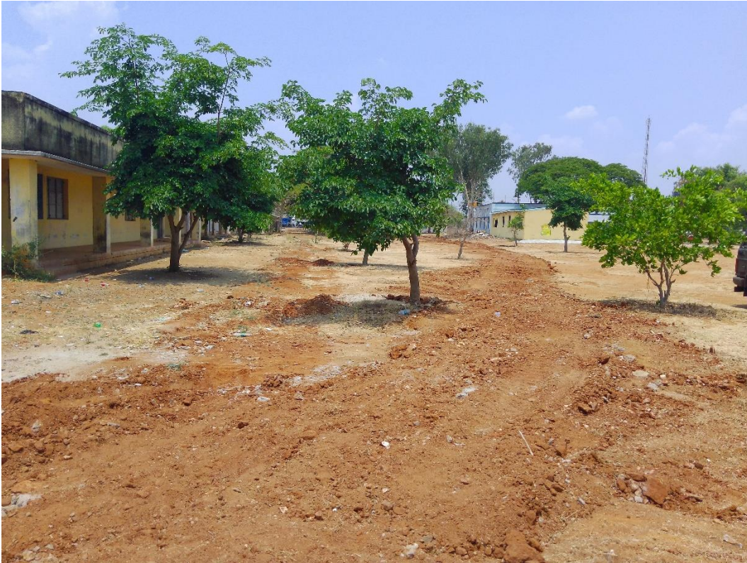
Water supply pipeline provided to Govt. High school and PU collage at Yaraballi village Hiriyuru Taluk
