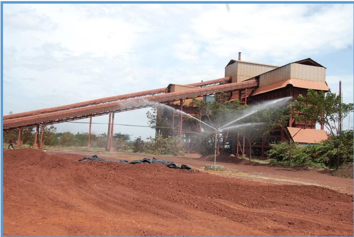
Sprinklers Installed at Mini Iron Ore Yard
