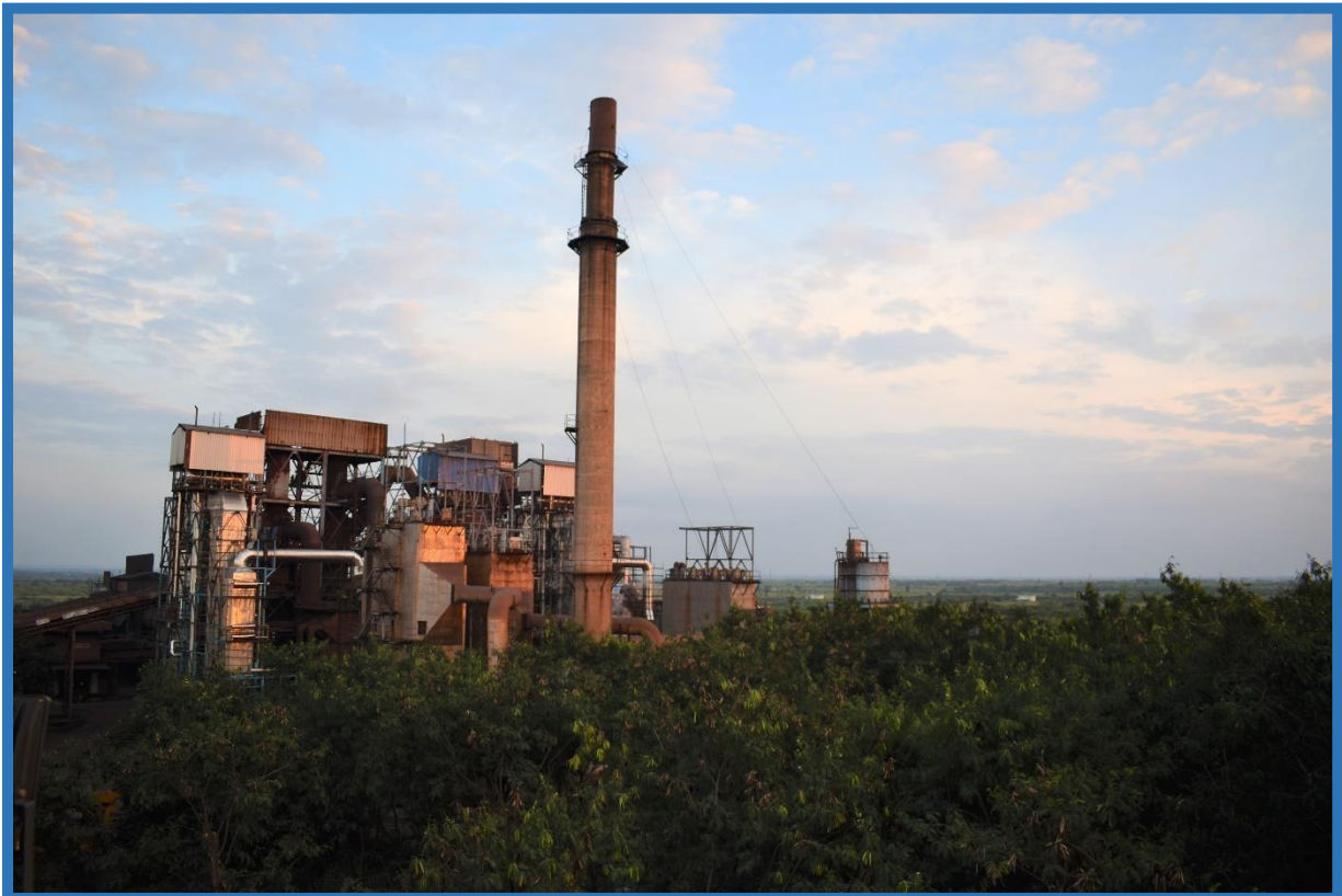
Air pollution control Equipment's with chimney
