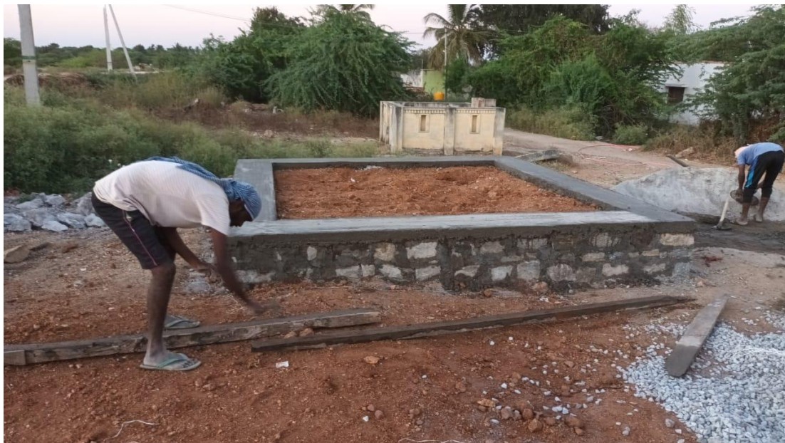
Construction of RO Water plant at Kaparahalli
