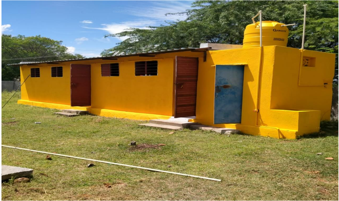
Construction of toilet block for GHP School at Heggere
