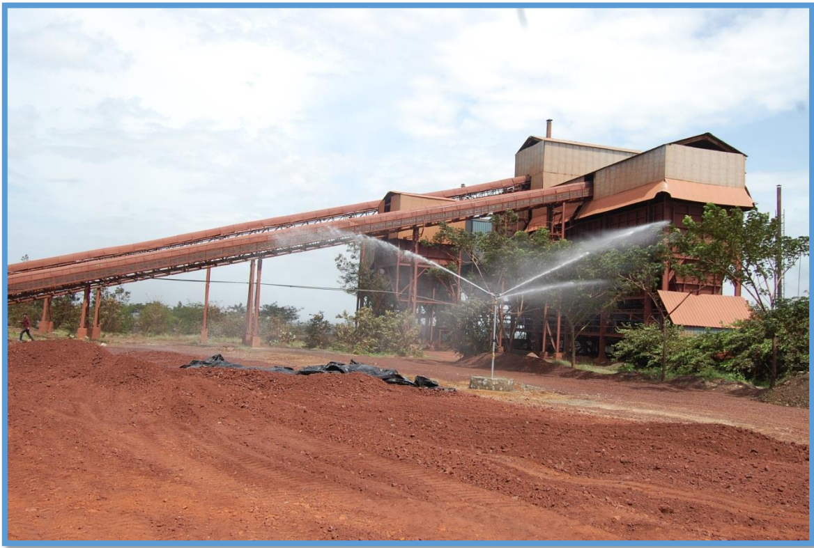
Sprinklers Installed at Mini Iron Ore Yard
