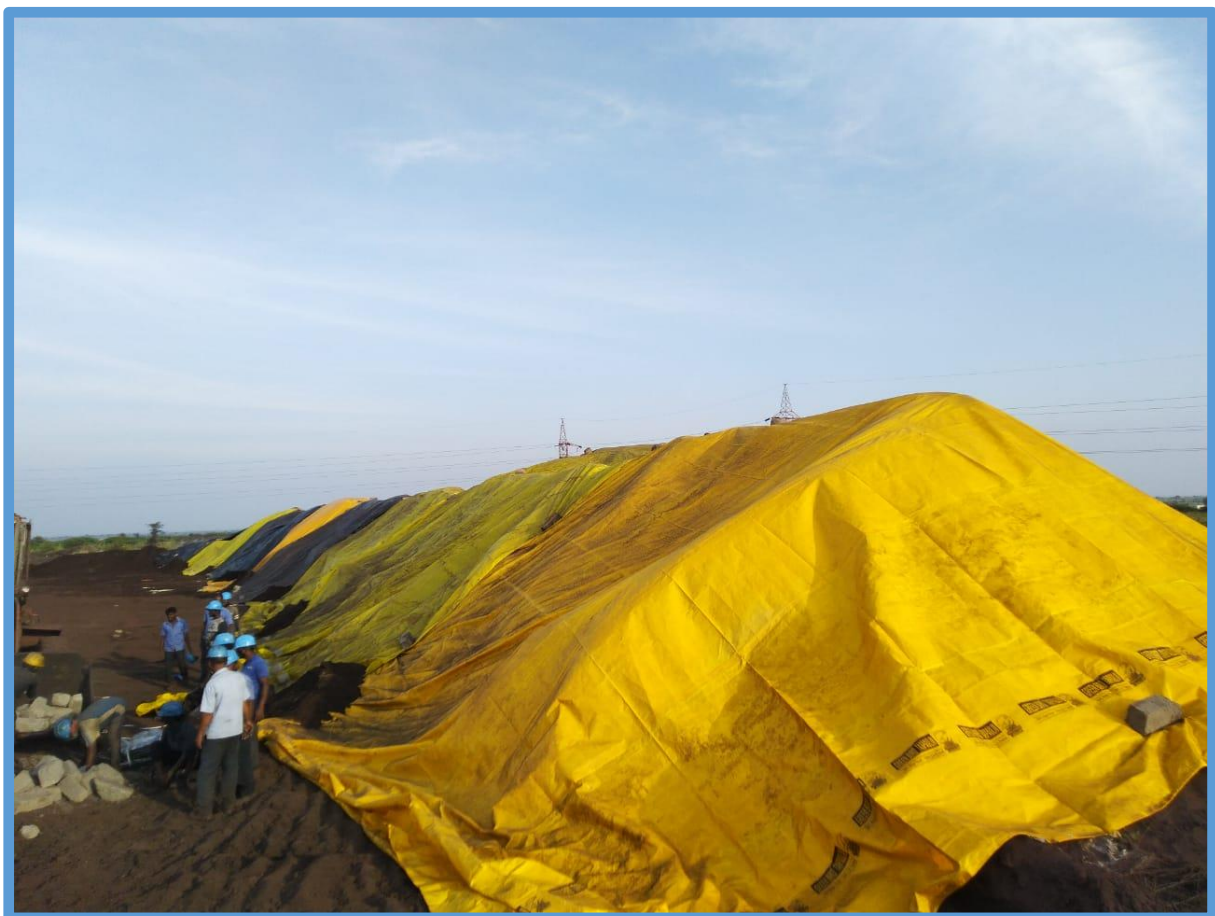
Covering of the Fly ash Dumps to Avoid Fugitive Emission.
