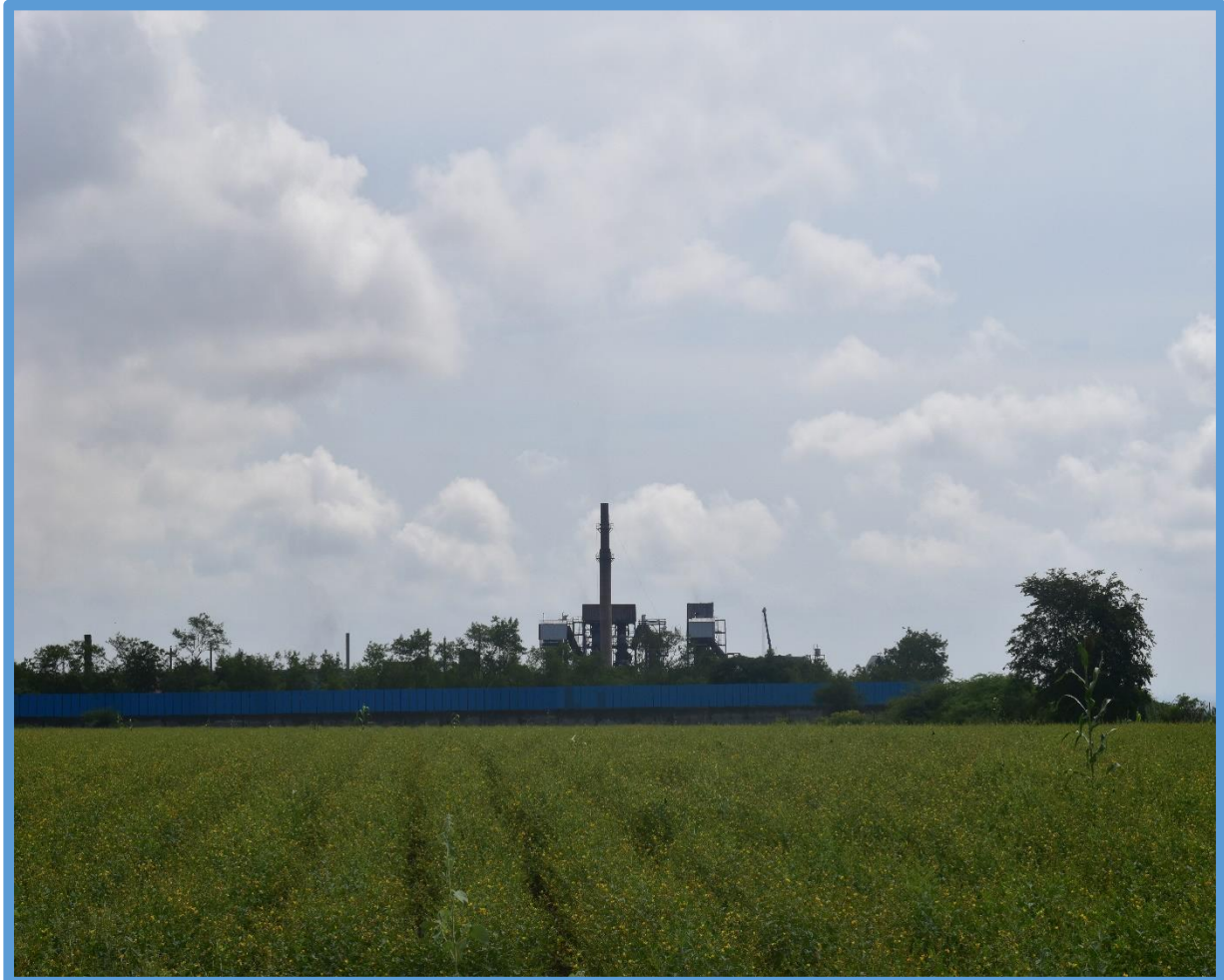
Air pollution control Equipment's with chimney
