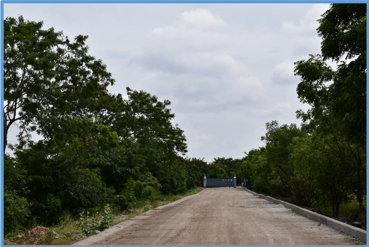
Concrete road with avenue Plantation
